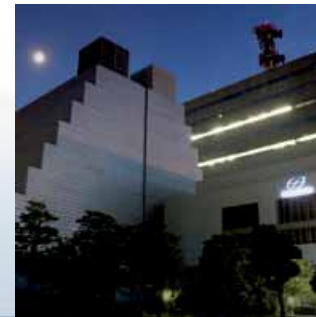
Combined heat & power plants (CHP)
